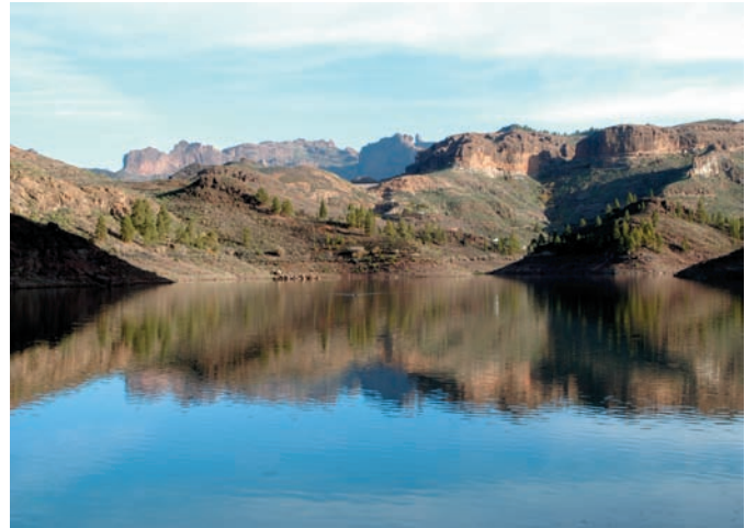
Top left: The Dam Wall at Chira. Above: Embalse de Chira.
